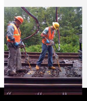
Specifically tailored with improved properties for cold weather application, ES-60 is manufactured to efficiently anchor spikes with comparable strength to un-spiked hardwood ties and is ideal for wood and composite railroad ties.
