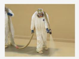
POLYQuik® P-480 is specifically designed to extend the service life of assets by protecting against corrosion, abrasion and concrete damage from a wide range of chemicals. This waterproof, polyurea coating can be sprayed directly to prepared steel and sets in seconds to form a virtually impenetrable barrier.
