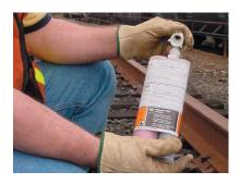
1. Unscrew the nut located on the top of the canister set and insert mix-tube through the screw nut. Set mix-tube with nut aside within reach.
