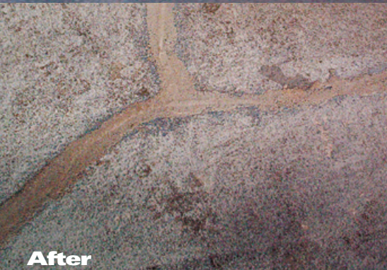
FastPatch LV fills cracks and levels to surrounding surface.
