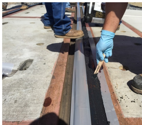
Figure 9: Leveling material.
