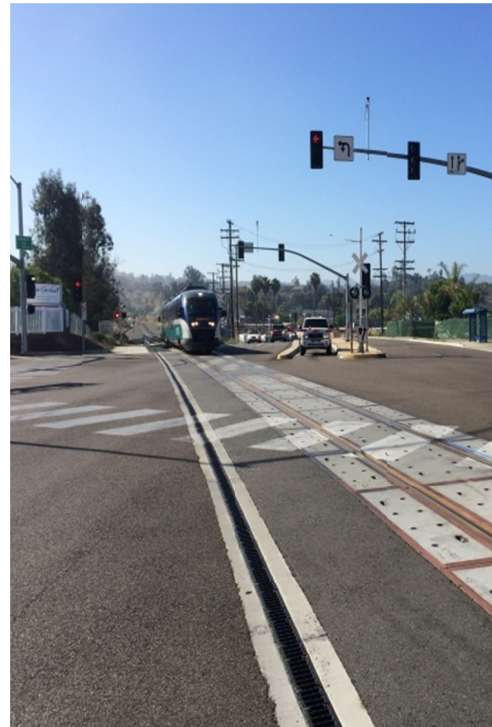
Figure 3: Track crossing for vehicles, pedestrians, wheelchairs, and bicyclists.
