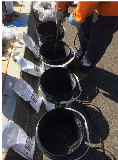
Figure 7: Staging material to fill gap on live track and traffic lanes.
