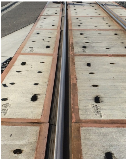
Figure 6: Hazardous field-side gap.
