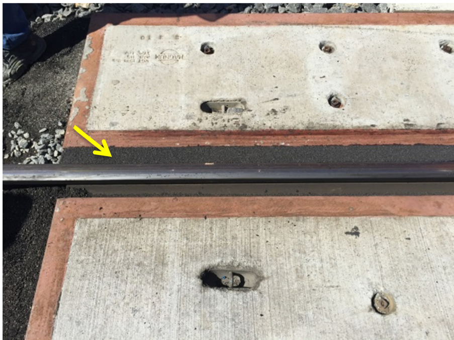
Figure 11: Filled gap with innovative material (AFTER).
