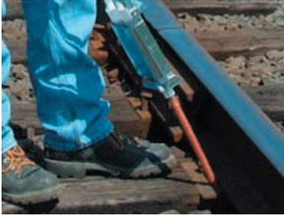
7. After filling mixing tube, immediately dispense SpikeFast into spike holes.
